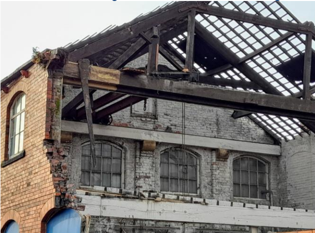
Demolition – nearing the end of the 1901 building. Note left the 'old overhead crane in situ amongst the rafters.
