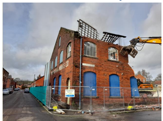
Demolition – nearing the end of the 1901 building. Note left the 'old overhead crane in situ amongst the rafters.
